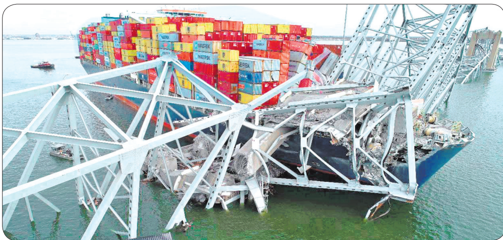
■ The Dali, with portions of the collapsed Key Bridge across its forward deck and in the Patapsco River, on March 28.
